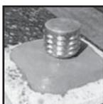
Terminate the flex by securely fitting the chosen Flue Factory terminal to the projecting section of the liner. Apply suitable acid resistant cement as a seal and
