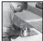
Secure and seal the liner to a debris plate, which closes off the appliance recess. Make sure that a little of the liner protrudes below the plate. Alternatively, the end of the liner can be sealed into the appliance flue pipe or socket on Flue Factory Flue Gas Collector, or Flue Box with non-combustible rope and/or fire cement.
