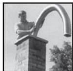
Attach the draw-cord to the nose cone. Use self-tapping screws to secure the nose cone to the end of the liner. Lower it into the chimney from the top, if necessary gently pulling from below using the draw-cord. When the lower end position has been determined remove the cone.
